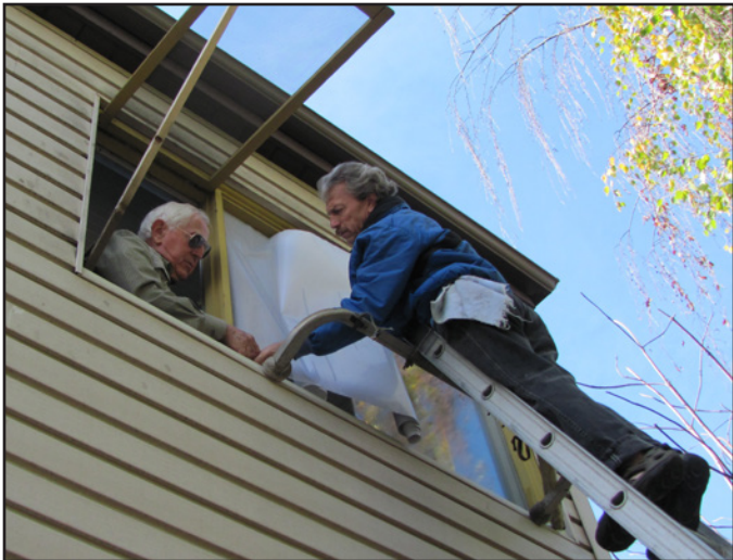
John Gaylord and Ken Vandehey install CollidEscape™ window film
